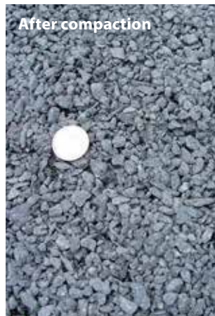
Fig 2. Chip seal pavement finished by GW750-2
