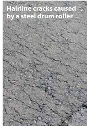
Fig 4. Remove hairline cracks from HMA pavement
