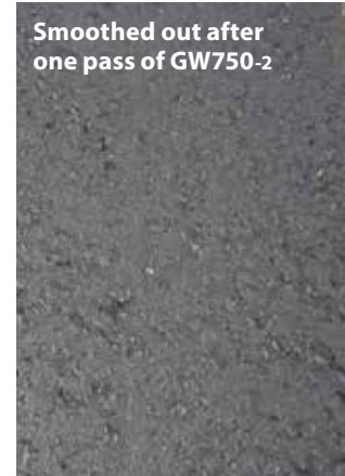
Fig 4. Remove hairline cracks from HMA pavement
