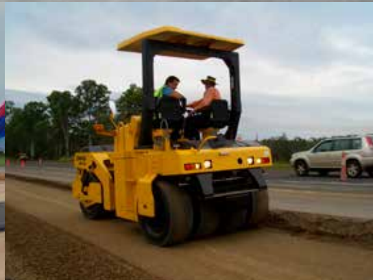
Soil subbase, Australia
